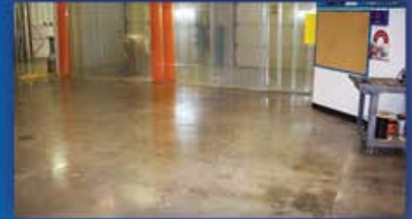
Warehouse Loading Area Cleaning
