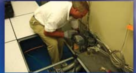
Access Panel Repair & Reconfiguration
