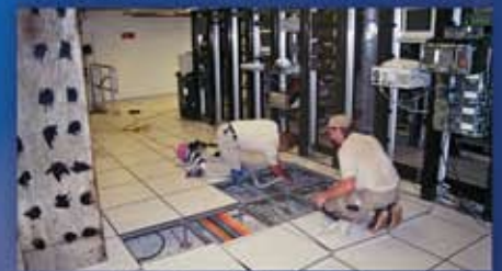
Computer Room Decontamination & Super Cleaning
